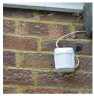
Here's a photo of the IR detector installed on an external wall of my house. Before you say it... Yes - I know having an exposed trailing cable is not "secure".
